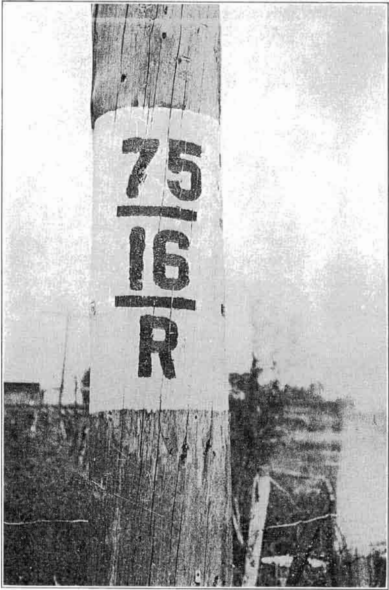
An illustration of the method used to Stencil Telephone Poles for the frequent information of travelers on Arkansas State Highways. This marking shows two roads overlapping, Nos. 75 and 16. The "R" indicates a right turn not far ahead.
