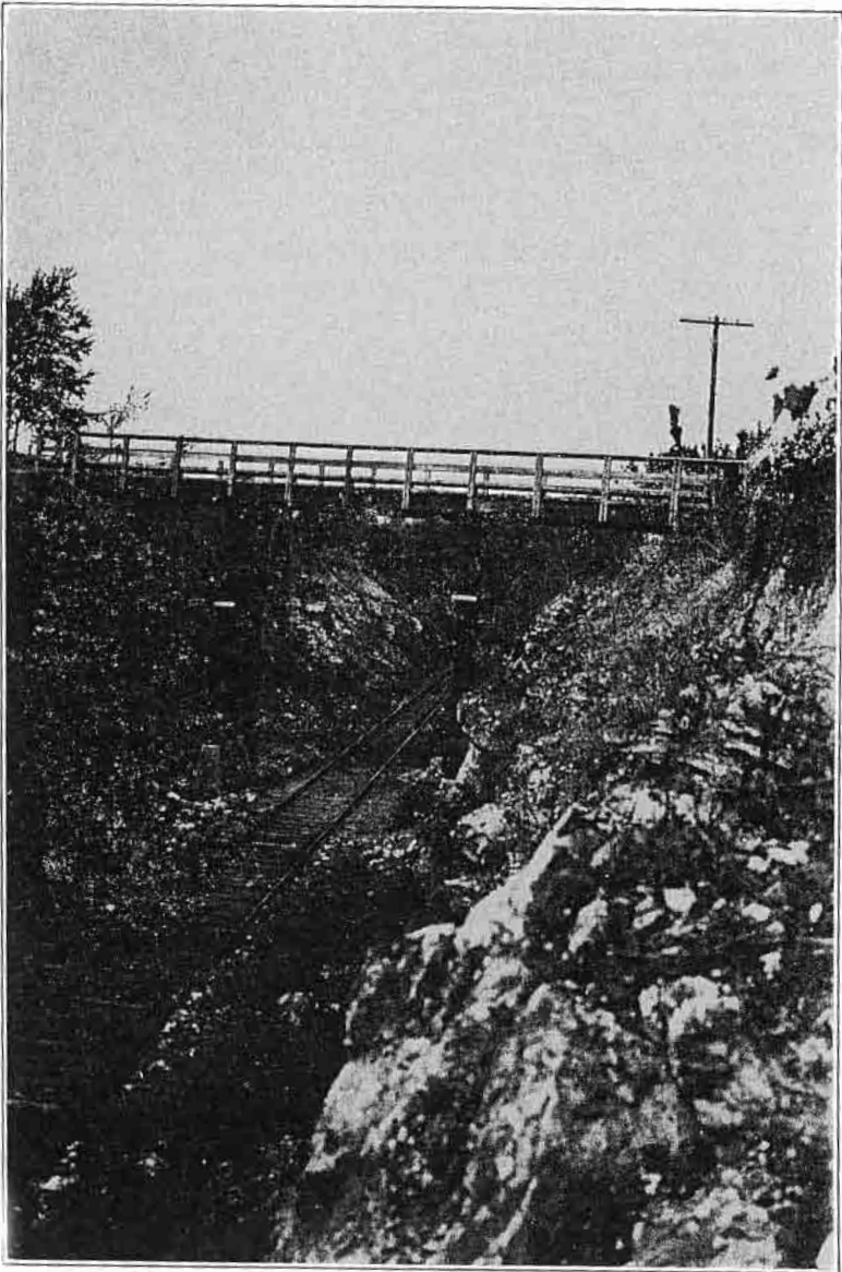
One type of grade separation work being done by the State in conjunction with the Railroad Companies. The crossing above is a Cresoted Timber Overhead Crossing of the Missouri Pacific west of Yellville in Marion County, recently completed and opened to traffic.
