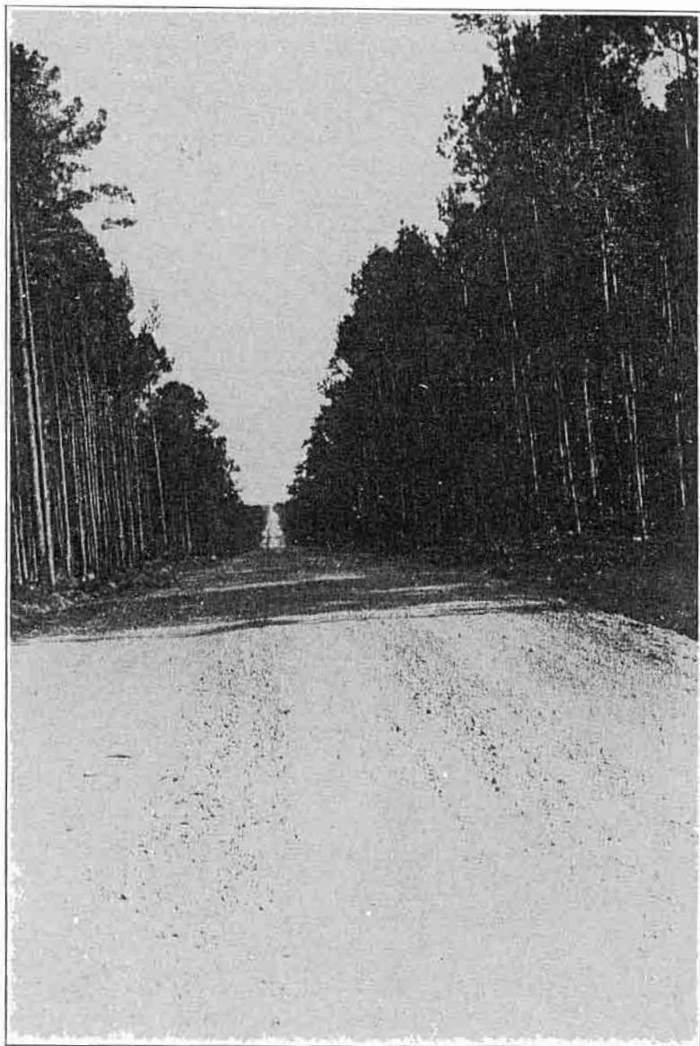
Federal Aid Project 225-A, El Dorado-Strong Road, Union County. An excellent Gravel Road completed in 1926.
